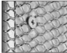
Wire lath to steel or wood studs.
